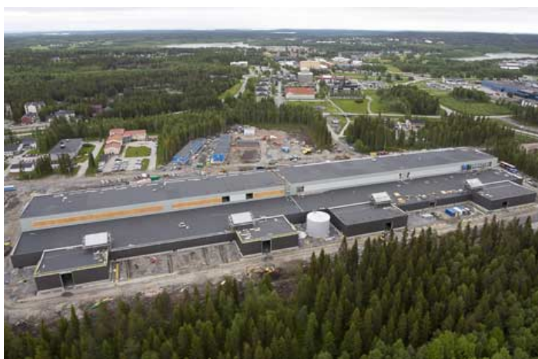
Figure 1.5: Aerial view of the Facebook datacenter in Luleå [5].
